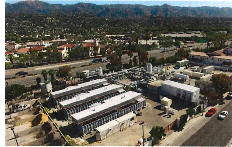
City of Santa Barbara, Charles E. Meyer Desalination Facility
