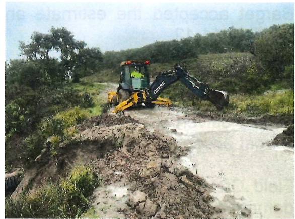
Temporary dam Mike Garner, District backhoe
