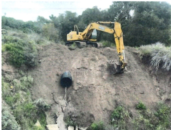
Reinforcing sewer main RL Johnson Construction
