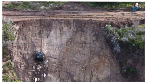
Work complete Sewer main reinforced, road restored
